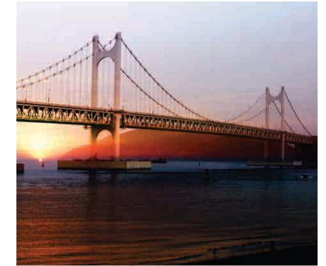
Gwangan Bridge • Location : Busan • Client : Busan City • Project Overview : - Total Length : 900m, Width : 25m - Type : Earthanchored Suspension Bridge
