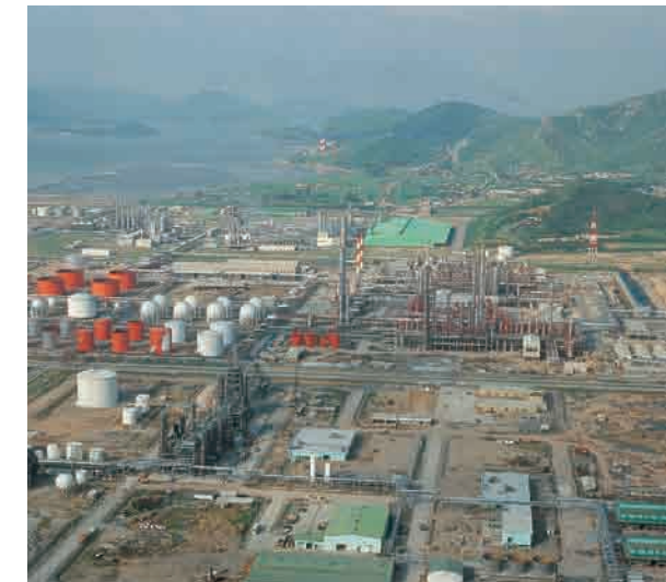
Ulsan Petrochemical Complex • Location : Ulsan • Client : Ministry of Construction
