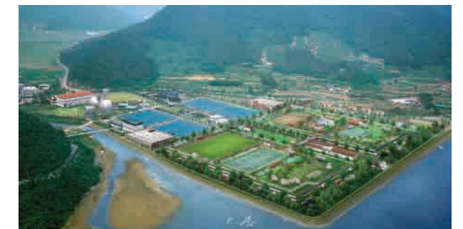
Deckdong Sewage Treatment Plant (Masan - Changwon Sewage Treatment Plant)
