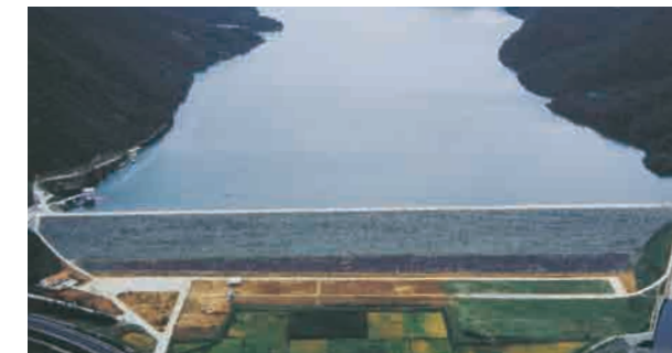
Jangseong Dam & Ancillaries
