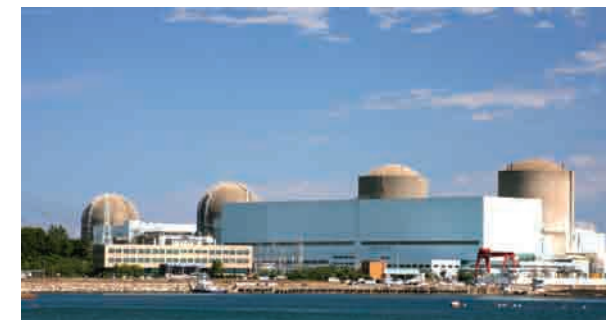
Kori Nuclear Power Plant No 1&2 • Location : Gijang-gun, Busan • Client : Korea Electric Power Corp. • Project Overview : 2 PWR Type Nuclear Power Plants with Capacity 600MW
