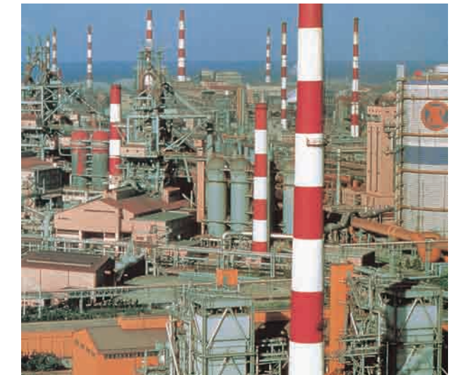
Pohang Steel Mill Plants Construction • Location : Pohang-si, Gyeongbuk • Client : POSCO • Project Overview : Steel Industrial Equipment Installation
