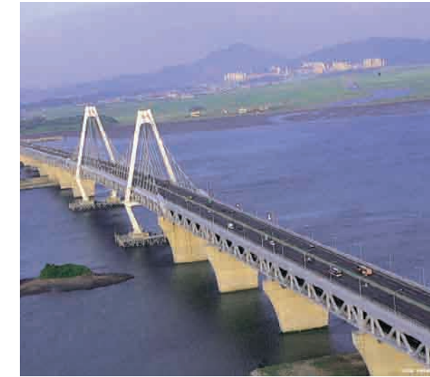
Youngjong Bridge • Location : Incheon • Client : The New Airport Hiway Co., Ltd. • Project Overview : - Total Length : 2,800m, Width : 36.3m - Type : Self-anchored Suspension Bridge / Warren Truss Bridge
