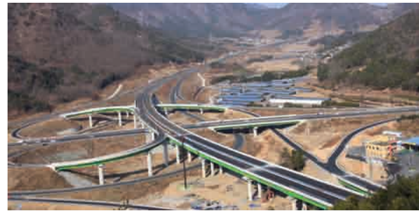
Hyungdong-Naeseo Road (4 lanes) • Location : Masan-si, Gyeongsangnam-do • Client : Busan Regional Construction and Management Administration • Project Overview : - Road : L=6,360m B=18.5m (4 lanes) - Bridge : 8 bridges/1,080m - Tunnel : Ssalijae Tunnel (L=1,465m)
