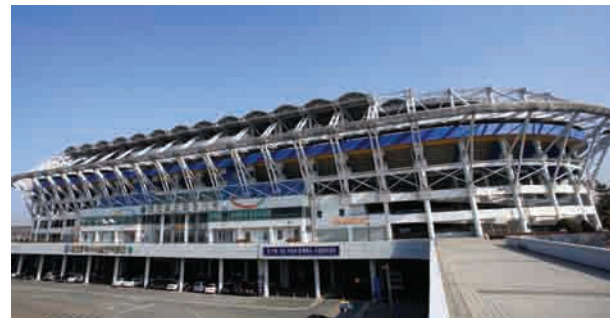
Daejeon Worldcup Stadium • Location : Yuseong-gu, Daejeon • Client : Daejeon Municipality • Project Overview : - 5 floors above and 1 underground, 42,176 Seats - Lot Area : 172,378,18m 2 - Building Area : 33,383,22m 2 - Gross Floor Area : 99,364.95m 2
