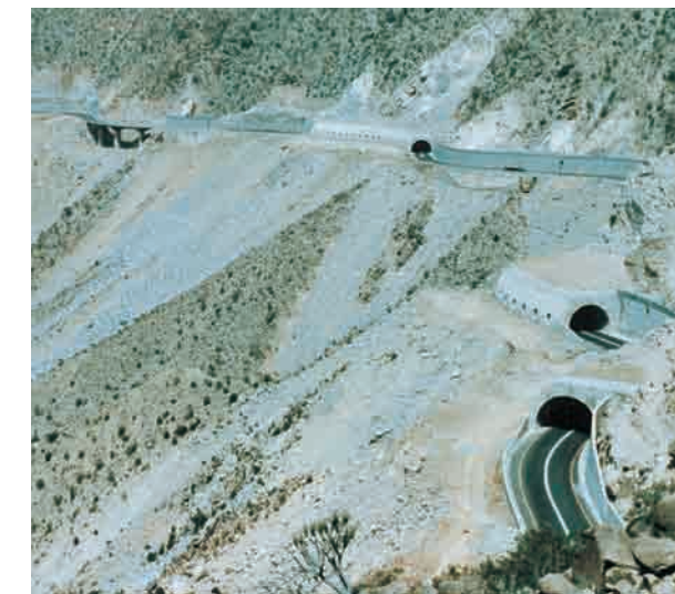
Al-Juwah Tihama Descent Road in Saudi Arabia • Location : Saudi Arabia • Client : Ministry of Posts, Telegraphs and Telecommunications (MOPTT) • Project Overview : - Length : 90km - Width : 11.6km - Tunnel : 30 EA (1,735m) - Bridge : 52 EA (3,764m)
