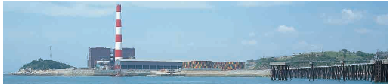
Seocheon Thermal Power Plant No. 1&2
