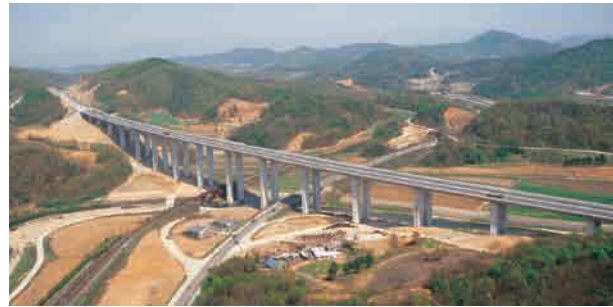
Jungang Expressway (wonju - Hongcheon) sec.17 • Client : Korea Highway Corp • Project Overview : - Road : L = 12.38km B = 23.4m - Bridge : 5EA
