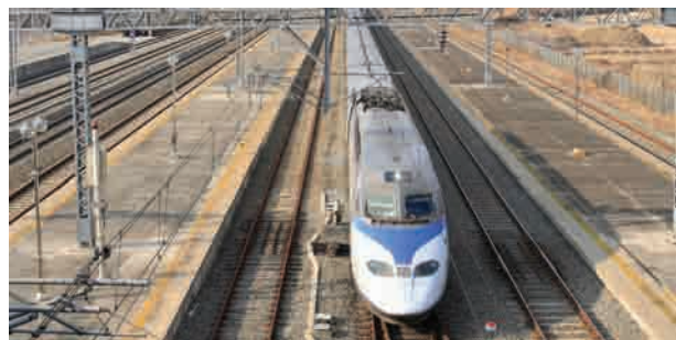
Relocation of Dongdaegu-Cheongchon Railroad • Location : The whole area of Hyomok-dong, Dong-gu - Gacheon-dong, Suseong-gu, Daegu • Client : Korea National Railroad • Project Overview : - Total Length : 7,800m - 5 Bridge : 56m (Palhyeon Bridge : Pront Jacking Method) - 2 Tunnel : 2 EA/540m - 3 Station : Gomo Station, Freight Station, Geumgang Station
