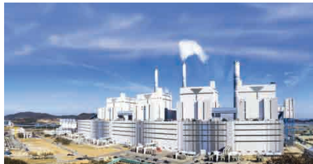
Yonghung Thermal Power Plant No. 1&2
