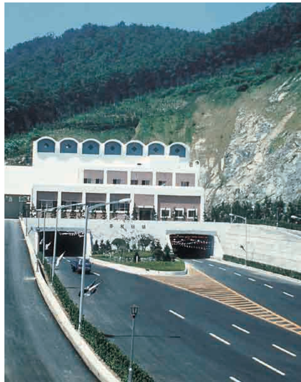
Kudeok Tunnel • Location : Seo-gu - Hakjang-dong, Buk-gu, Busan • Client : Busan Municipality • Project Overview : - Total Length : 1,870m (NATM) - Radius: 4.7m, Section Area 62.3m 2
