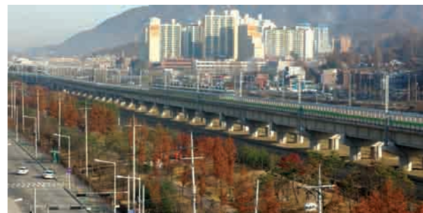
Kyungwonseon (Eujeongbu-Dongducheon) 2-track Line • Client : Korail • Project Overview : - L=7,948m, Earthwork: 266,379m 3 - Bridge: 3 EA (L=5,177m) - Station: 5 EA
