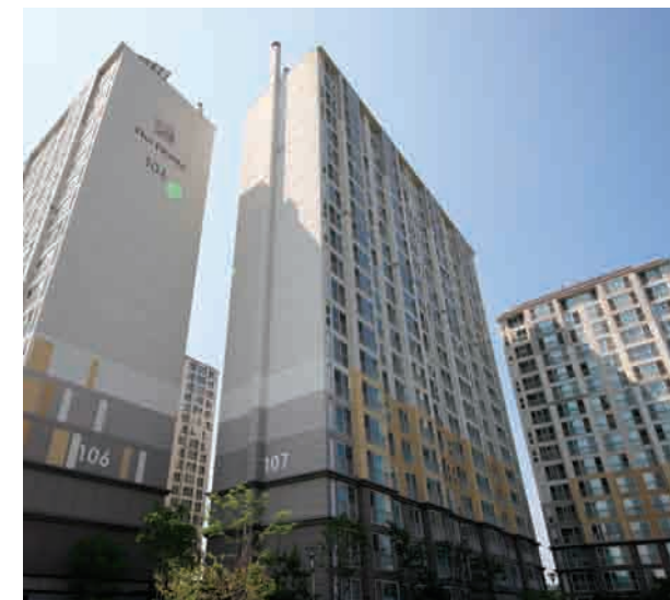
Changnyeong Namji The PRIME Apartment
