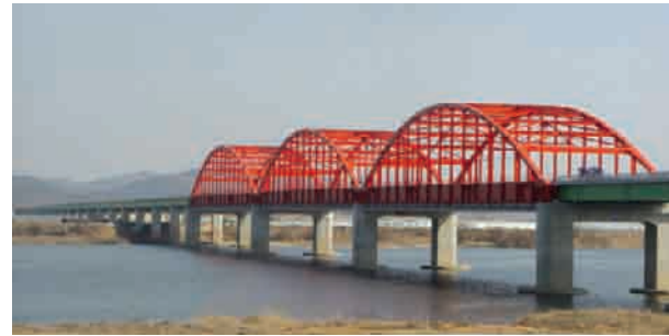
Kuryong - Buyeo Road Expansion • Client : Daejeon Regional Construction & Management Administration • Project Overview : - L=8.40km, B=20m - Bridge : 1 EA (L=1,595m)
