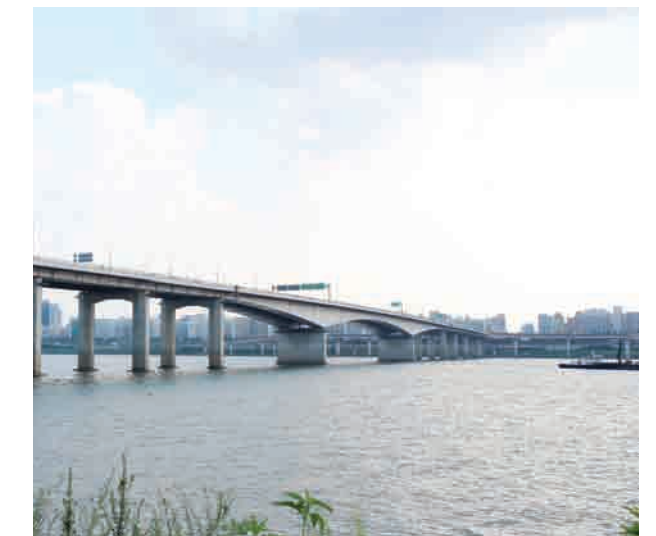
Gayang Bridge • Location : Seoul • Client : Seoul Metropolitan Government • Project Overview : - Total Length : 1,603m, Width : 16-29m, Span Length : 180m - Type : S.T BOX Girder
