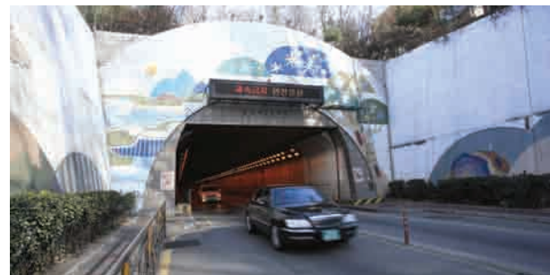
Namsan Tunnel Line No. 2 • Client : Seoul Metropolitan Government • Project Overview : - Length = 1,680m
