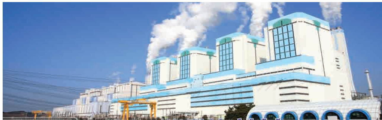
Dangjin Thermal Power Plant No.1&2
