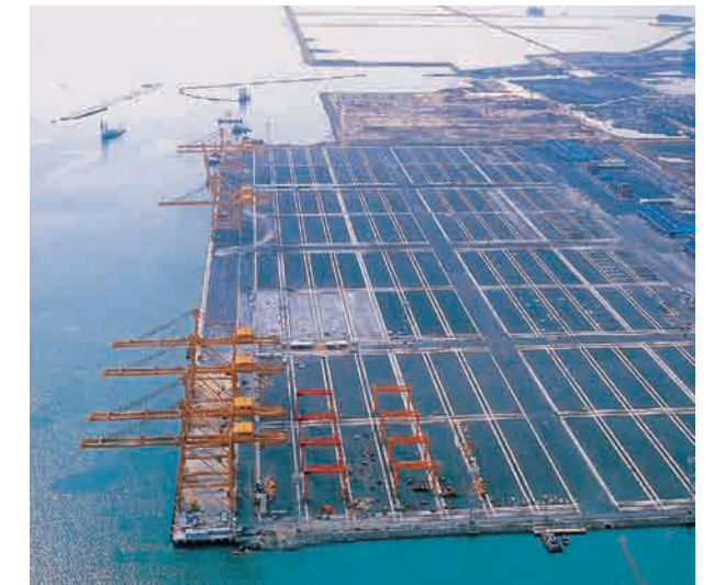
Gwangyang Port Container Terminal • Location : The Sea around Doi-dong and Hwanggil-dong, Gwangyang-si, Jeollanam-do • Client : Korea Container Terminal Authority • Project Overview : - Container Terminal 50,000 DWT - Caisson Manufacture and Installation : 108 Cases(L=1,144.8m) - Crane Rail Laying : 2,760m - Pavement Work : 8,478a - Construction Work : 43 buildings(except operation building) - Electric Pipelining Work : 10,450m
