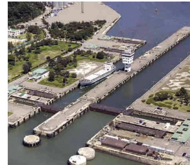
Gate Expansion for Incheon Port • Location : The whole area of Incheon Inner Harbor 80-9, Bukseong-dong 1-ga, Jung-gu, Incheon • Client : Incheon Regional Maritime Affairs & Port Office • Project Overview : - Floodgate Facility 10,000 ton - Caisson Manufacture 24,166 ton - Door Manufacturing and Installing : 488.58m 2 - Shore Protection : 29.32m - Mooring Facility : Wharf for Samll Ship 136.5m - Dredging : 138,761m 3
