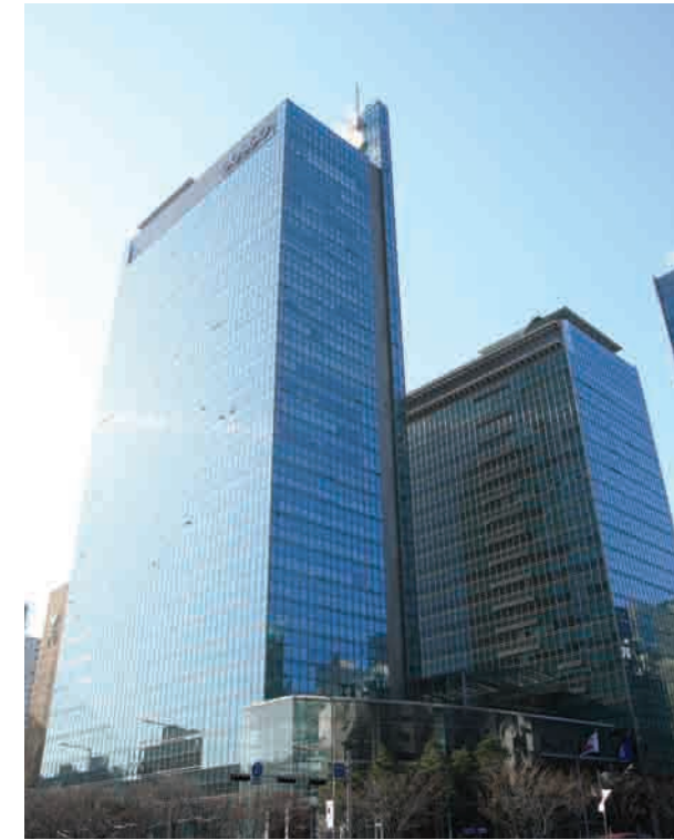
POSCO Center • Location : Gangnam-gu, Seoul • Client : POSCO • Project Overview : - High-tech Information-orientated Building (20-30 floors above and 6 underground) available for 4,500 people - Lot Area : 17,454m 2 - Building Area : 7,305m 2 - Total Floor Area : 181,587m 2
