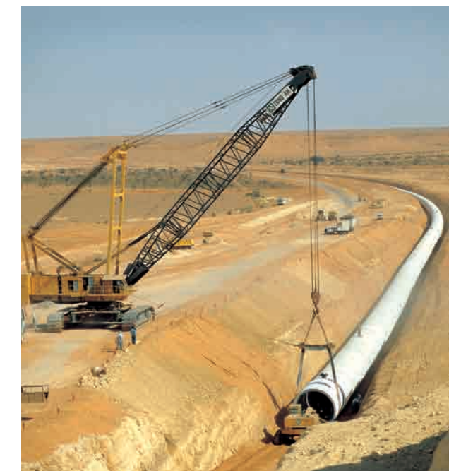
PCCP Laying & Transportation
