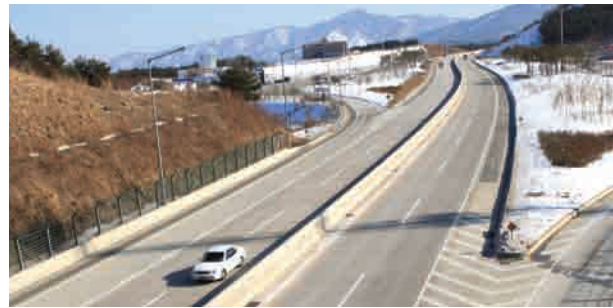
Donghae-Jumunjin Highway Expansion • Location : Gangneung-si, Gangwon-do • Client : Korea Highway Corp. • Project Overview : - Road : L=5,109m, B=23.4m (4 lanes) - Bridge : Long-spanned Bridge (4 spots/2,797m) - Namdaejeon Grand Bridge : L=1,041M (FCM+LLM) - Construction : Gangneung Branch and Gujeong Resting Place
