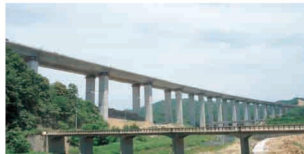
Yeongdong Expressway (Singal - Wonju) Expansion • Client : Korea Highway Corp • Project Overview : - Road : L = 5,056m B = 23.4m (4 lanes) - Bridge : 780m (1.L.M Method)
