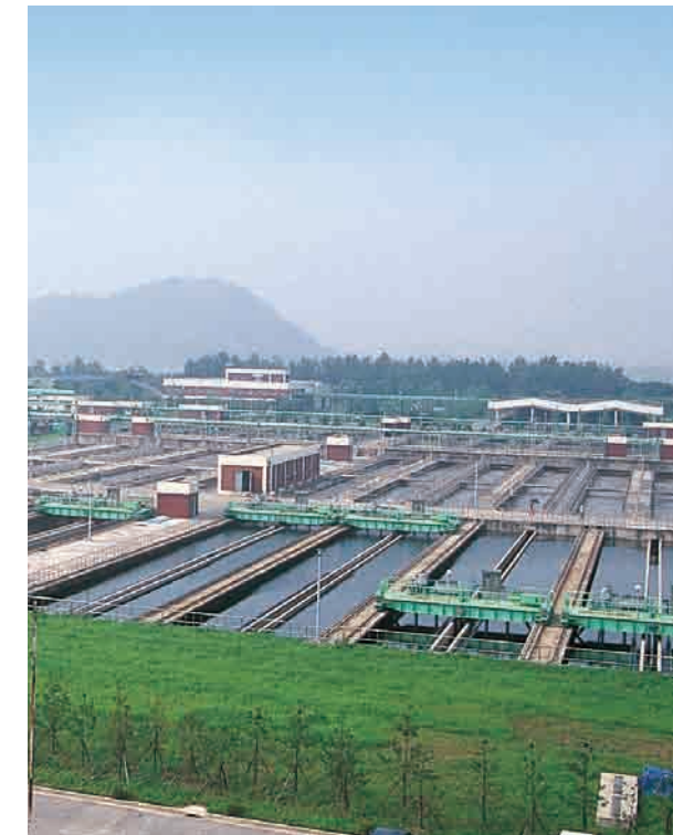
Kayang Sewage Water Treatment Plant Expansion
