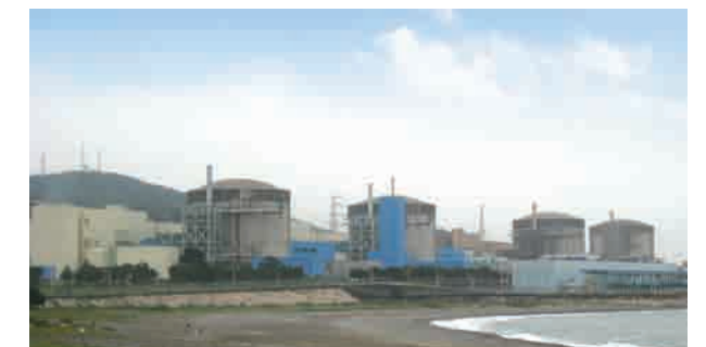
Wolsong Nuclear Power Plant No. 1 • Location : Gyeongju-si, Gyeongbuk • Client : Korea Electric Power Corp. • Project Overview : 1 PHWR Type Nuclear Power Plant with Capacity 650MW
