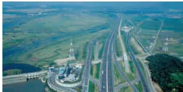
Incheon Int'l New Airport Road & Bridge • Location : Incheon - Unbok-dong, Jung-gu, Incheon • Client : New Airport Highway Co., Ltd • Project Overview : - Express : L=3,830m B=36.3m (6 lanes) - Bridge : Truss Bridge L=250m / Steel-concrete Composite Bridge L=450m - Railroad : L=250m (double-track)
