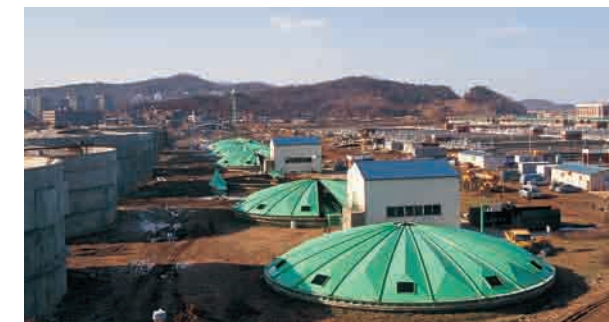
Anyang River Sewage Treatment Plant
