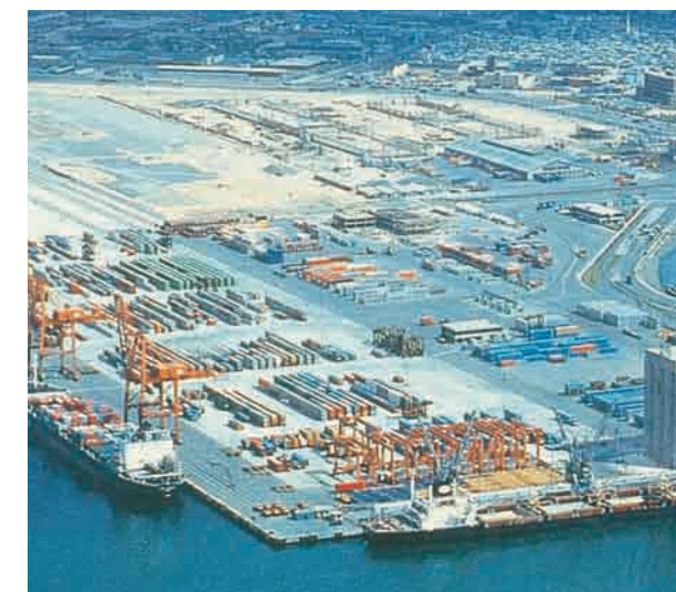
Busan Port No. 3, 4, 7, 8 • Location : The Sea around Doi-dong and Hwanggil-dong, Gwangyang-si, Jeollanam-do • Client : Korea Marine & Port Administration • Project Overview : - Capacity : 1,000 - 15,000 DWT (10 Berths) - Reclamation : 2,107,400m 2 - Dredging : 1,070,000m 3 - Paving : 166,600m 2
